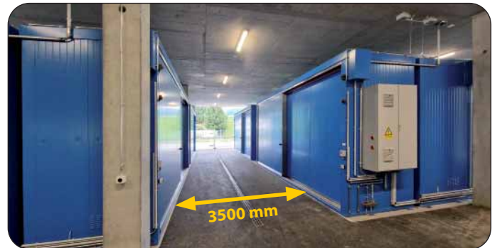
◆ Small aisle width due to the use of sliding gates
