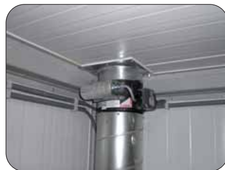
Air exhaust duct with K-90 shut-off device
