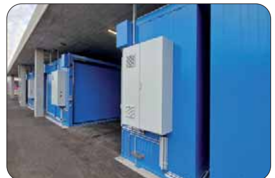
◆ Small aisle width due to the use of sliding gates
