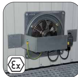
Technical forced ventilation, ex-proof, Article no. H61-9006-C
